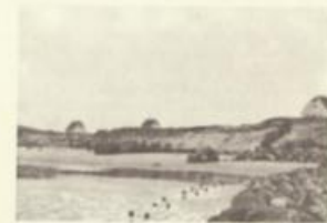
Fig. 19. The leeside-groin at the Old Skaw.
