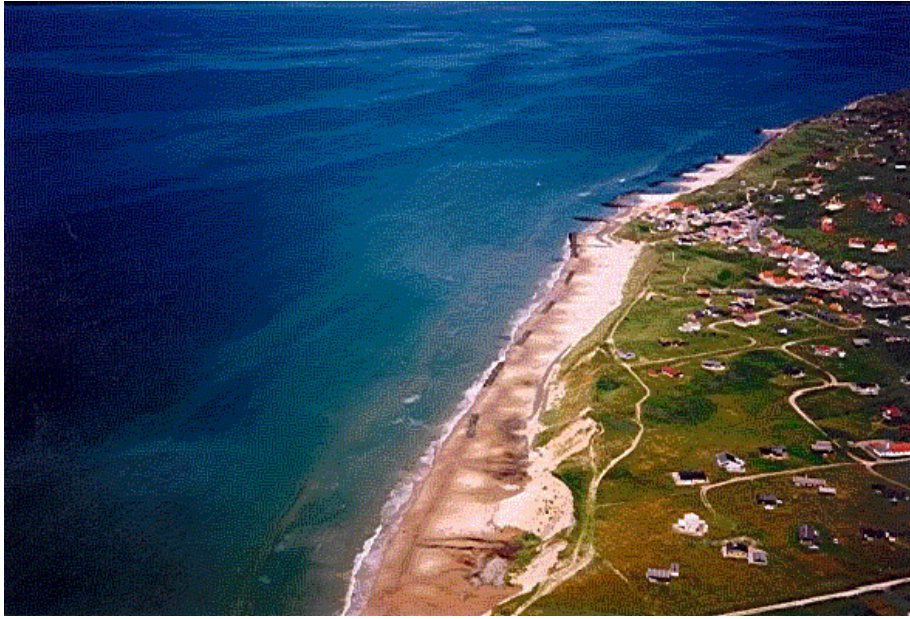
Fig. 13 Lønstrup after PEM installation 1999
