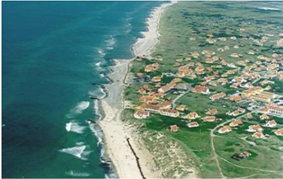
Fig. 11 Gl. Skagen PEM installation removed in 2001
