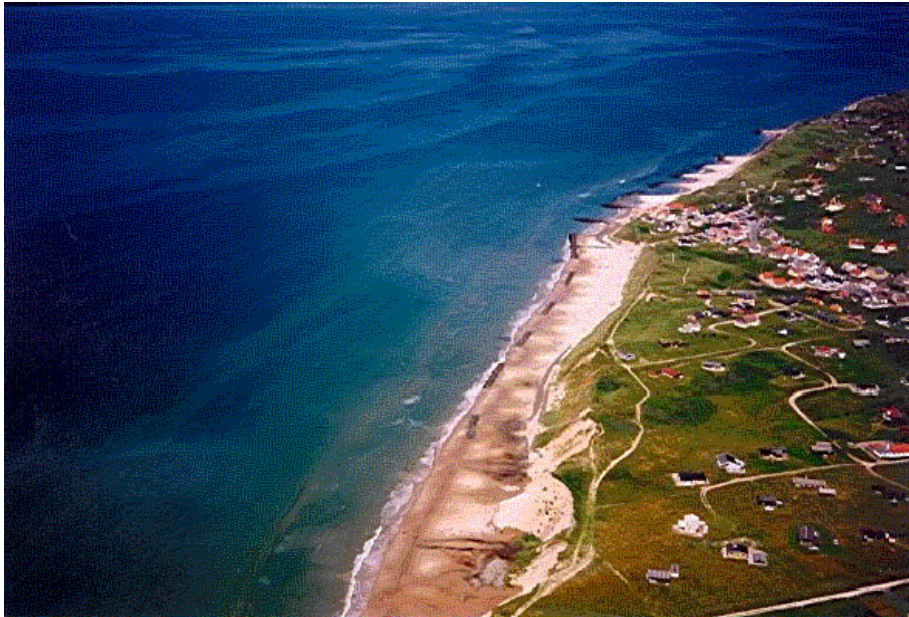
Fig. 13 Lønstrup after PEM installation 1999
